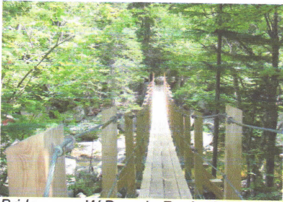
Bridge over W Branch, Peabody River, NH. By Mike Calabrese
